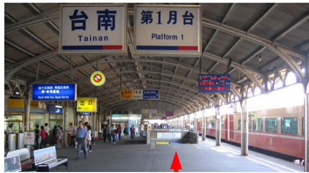
Go to the rear exit of the station through the underground
